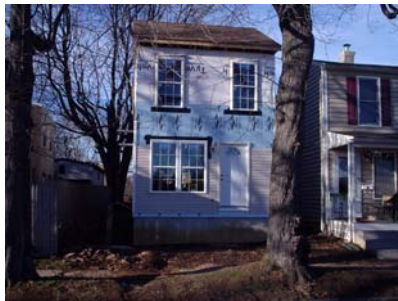
Picture of home under construction at 427 East Barnard
